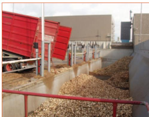
Container truck delivering chips to the chip reception pit of a large co-generation plant.
